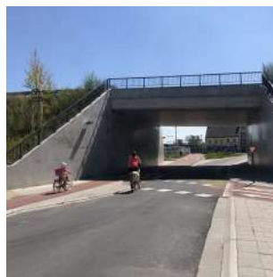
Tunnel richting station
